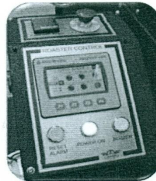
BPR OPERATING PANEL
