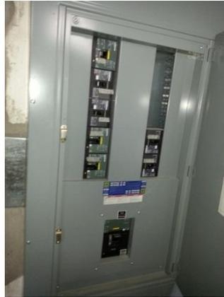
**Figura 16. Tablero Principal Schneider Electric**
