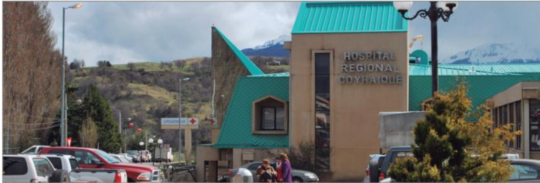
Figura 12: Hospital Regional Coyhaique
