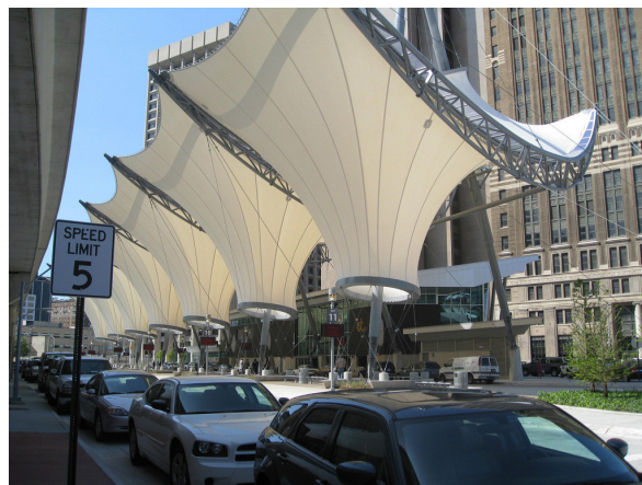
Centro de Tránsito Rosa Parks, FTL Design Engineering Studio
