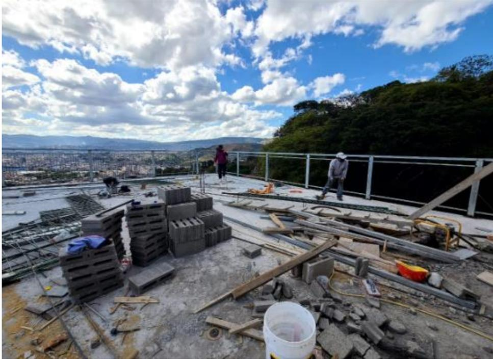
**Ilustración 304 Continuation of installation of railings**
