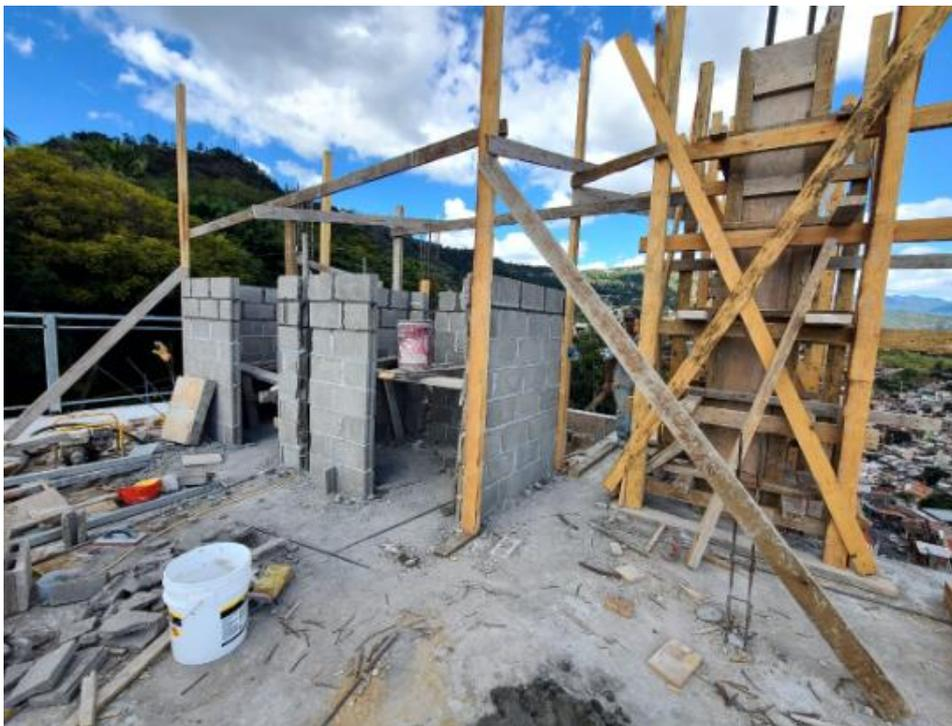
**Ilustración 305 Continuation of construction of walls on rooftop**
